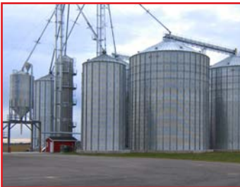
Grain Storage Bins
