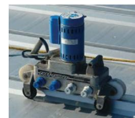
The seaming process uses a heavy-duty four-stand, electric, portable roll-forming machine called the Roof Runner.
