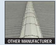
Butler's minimal use of exposed fasteners not only reduces the potential for leaks but also saves on installation costs. Additionally our exclusive Lock-Rivet™ fasteners with factory-punched holes eliminates the need for drilling. This eliminates the metal shavings which cause rusting as found in other manufacturers' ridge designs.
