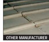
**Above Top:** Butler staggers panel splices to avoid the four-corner condition—another design feature to assure weathertightness and longer roof life.
